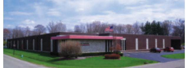
Carson Manufacturing Company, Inc.'s headquarters and 47,000 square foot manufacturing facility located in Indianapolis, Indiana.
